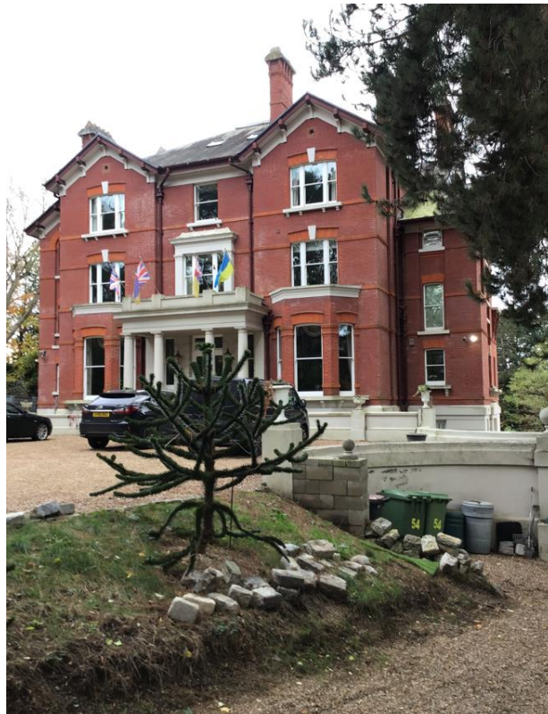
Figure 4: Photograph of No.54:
