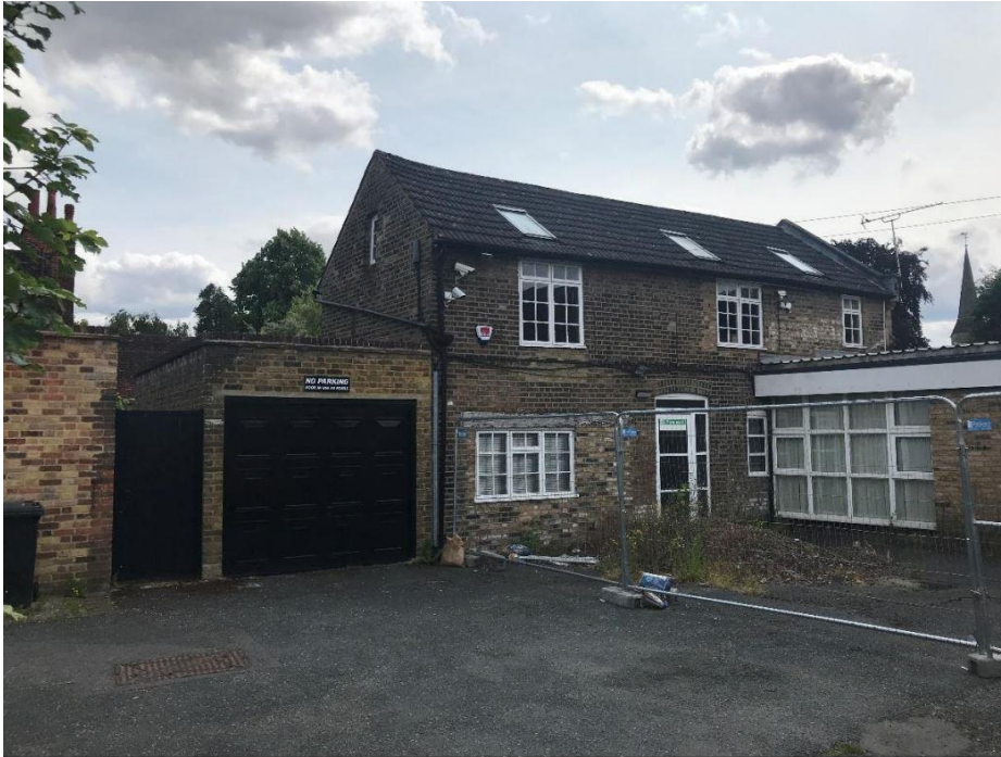
Photograph 3 internal site looking south east.
