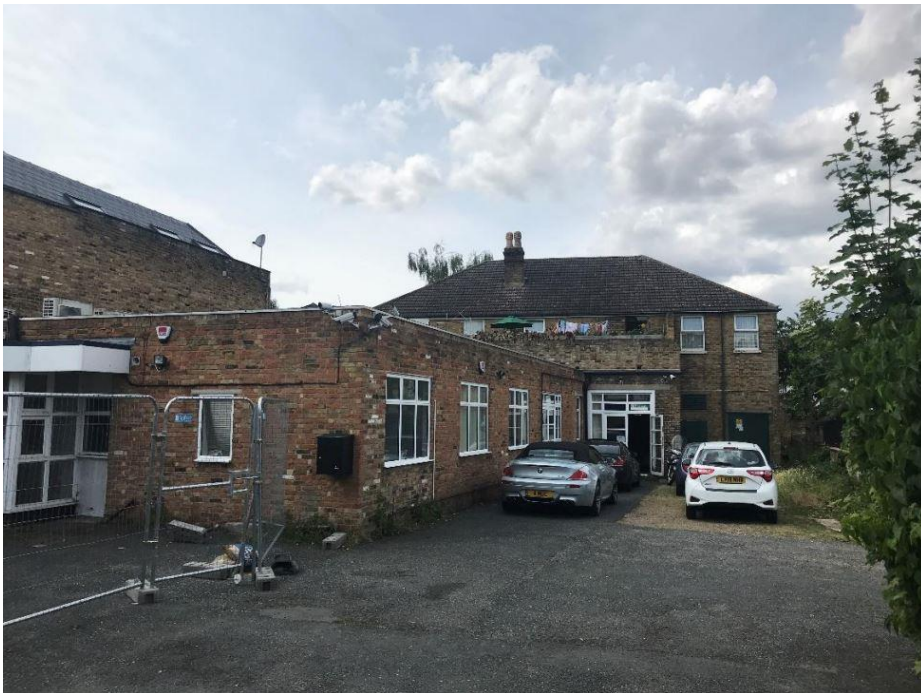
Photograph 4 internal site looking northwest towards existing maisonette.
